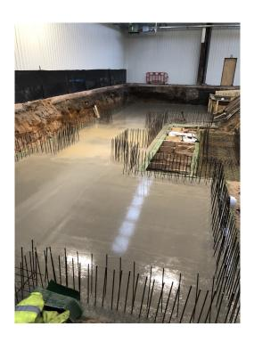
Middle right of the picture is where the u-pit will be formed. There is additional strengthening to be added then the shutters will go up and then more concrete to be poured, forming the pit walls ready for the fit out by Gymnova in February.
